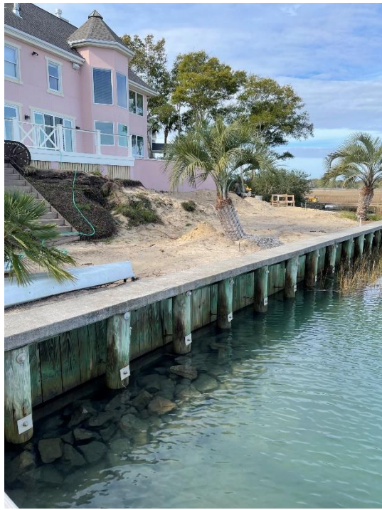
013-timber bulkhead, 3 WWI, construction work underway
