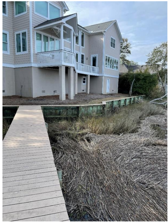
014-timber bulkhead, 4 WWI, conditions unchanged since 2021 inspection
