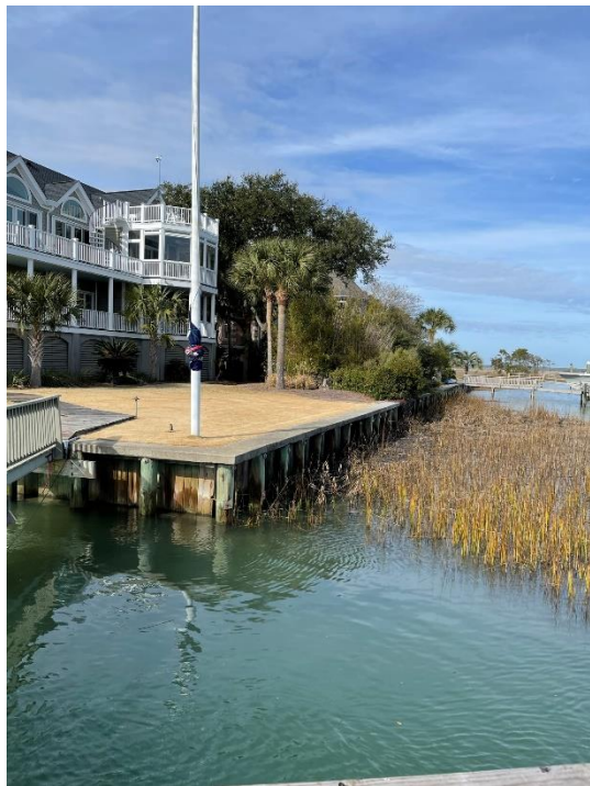
011-timber bulkhead, 2 WWI, conditions unchanged from 2021 inspection
