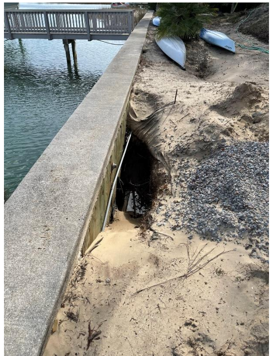
012-timber bulkhead, 3 WWI, landscaping and repair of backfill subsidence in progress
