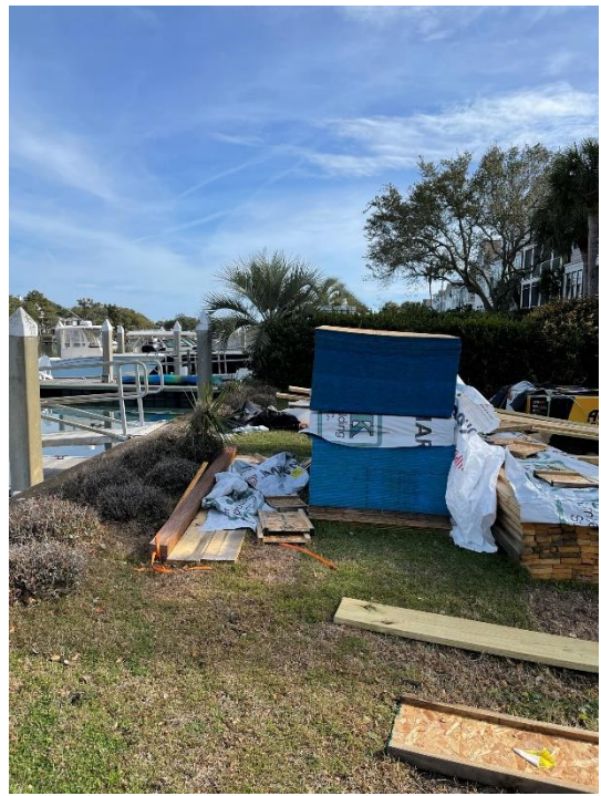
008-stockpile of construction material near the wall Station 36+00
