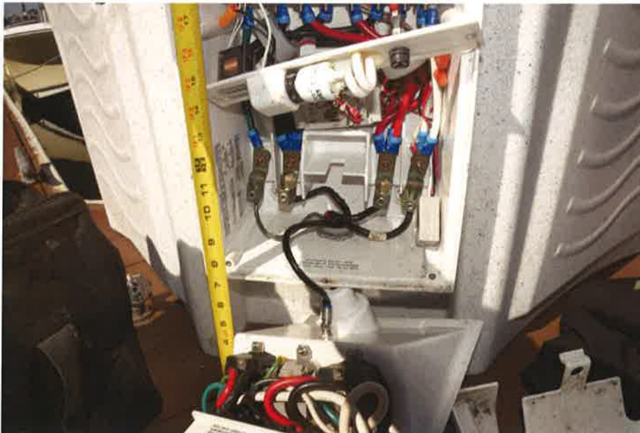
Dock box mounted pedestals
